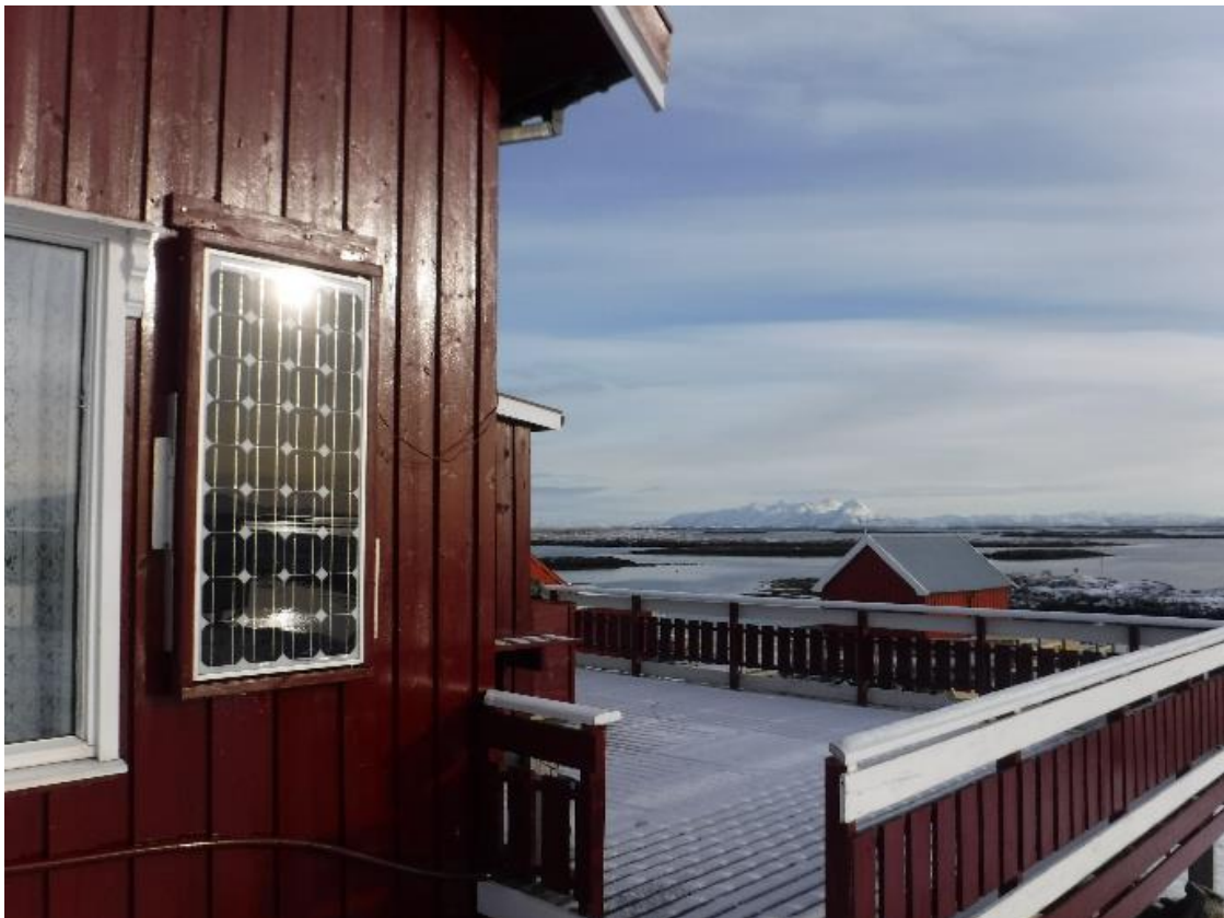
Mains electricity is not available on most islands and solar panels are frequently used on placed like Lånan - 21 February 2017 ©IUCN/Colin Bean
