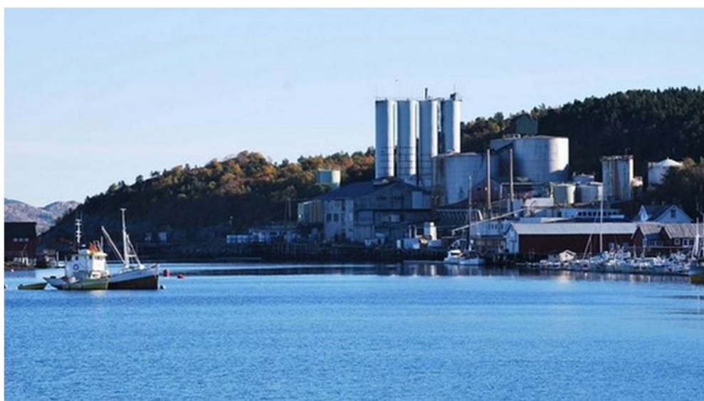
(Scanbio AS fabrikkannlegg i Lysøysundet)
