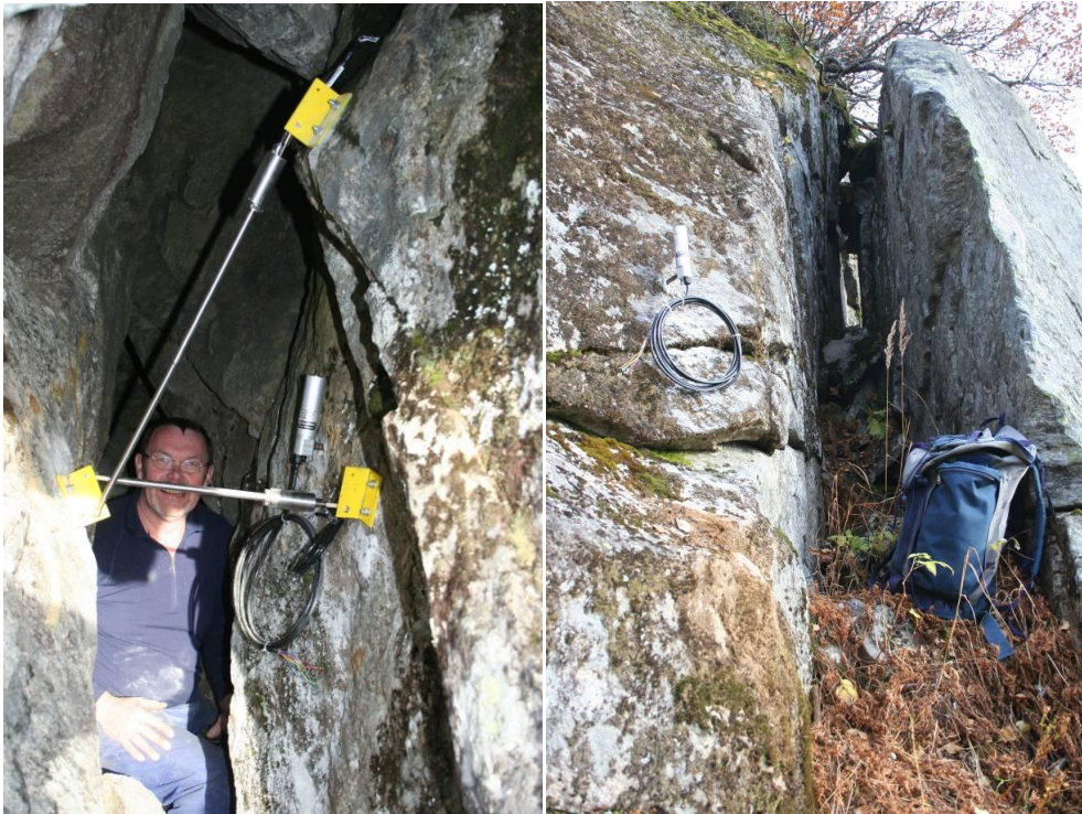
FIGURE 5: CRACKS AND INSTALLATION OF CRACKMETERS AT HEGGURAKSLA.
