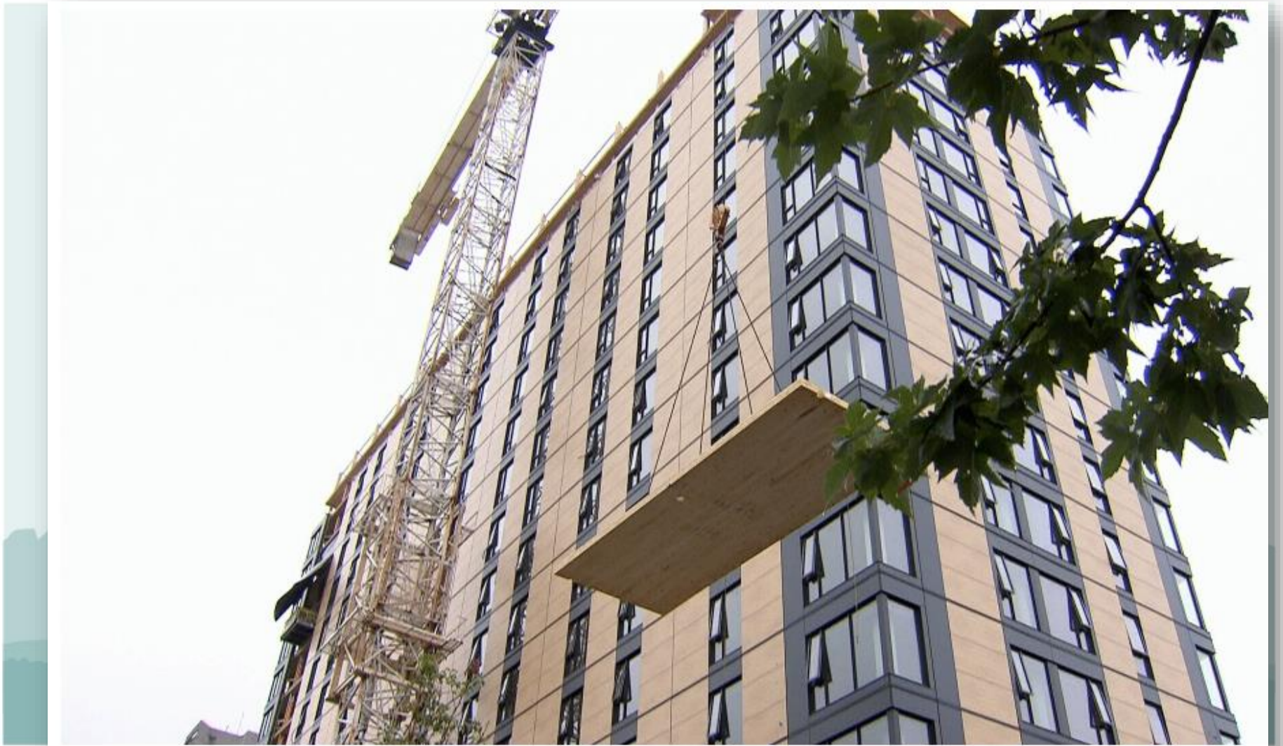
The final wooden panel was put in place on Tuesday, Aug. 9, 2016.
