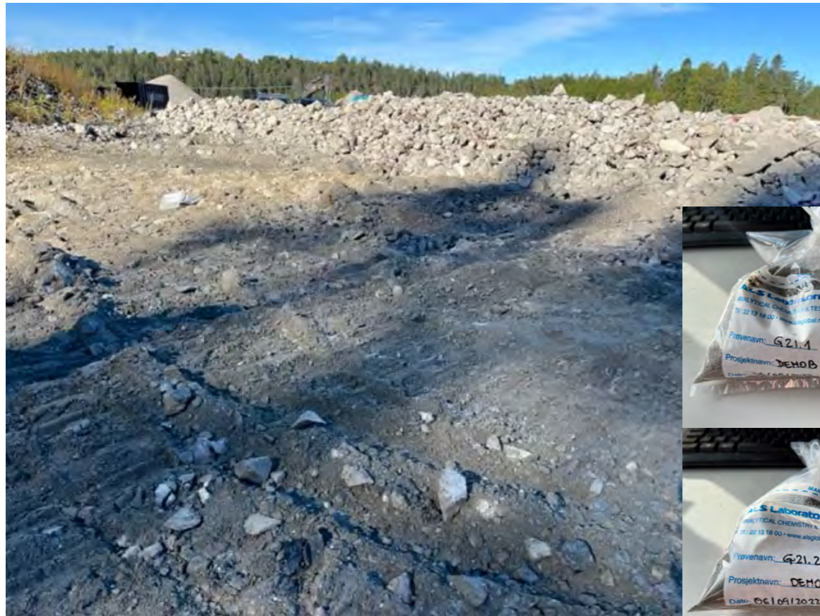
Sample: G21 Concrete point
