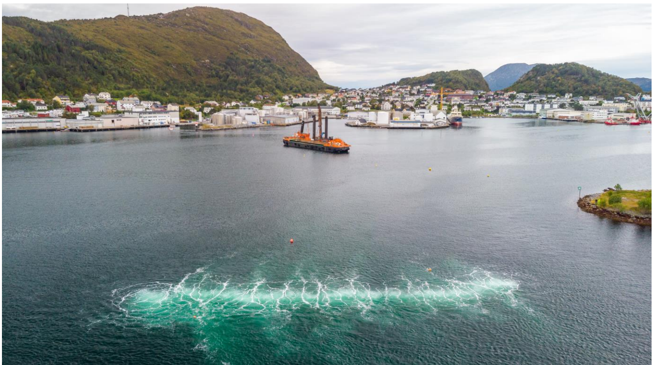
Figure 6: Bubble curtain in line configuration in the foreground and blast location (Source: Kystverket)
